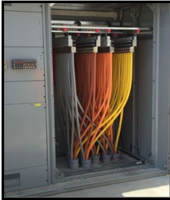
Color coded 277/480V phasing example with colored secondary conductor installation.
